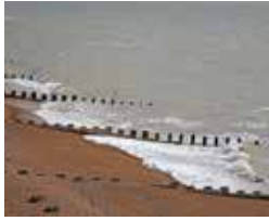
Figure 4.13 Various structures are built on beaches to prevent erosion due to longshore transport.
